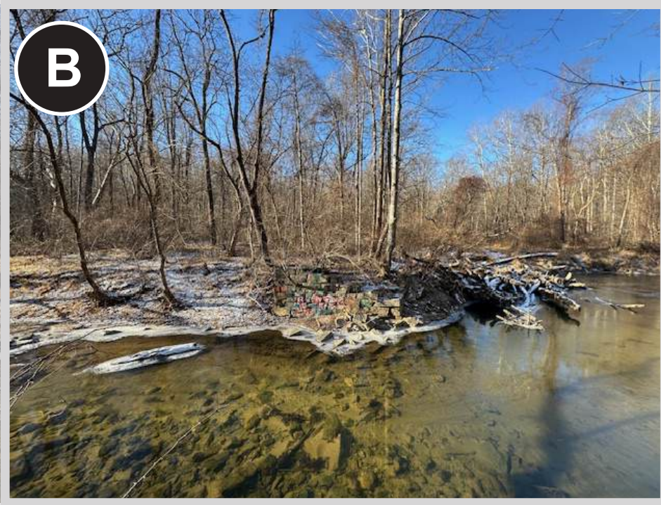
Looking south to former bridge abutment on Edinbrook side of river. Crossing Location B.
